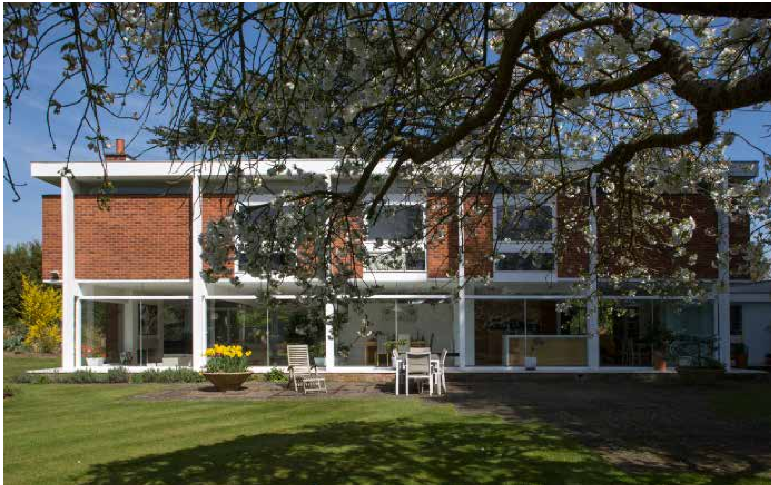
Cedar Leys in 2015. Womersley's logic is consistently applied in the rectangular plan, the elevations offering a 'faithful reflection' of the inner programme through apparently floating panels of hand-made brick at the upper floor and single glazed sliding units to the south-facing facade
