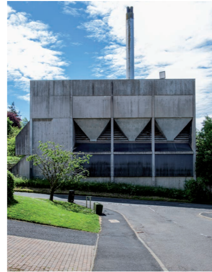
Dingleton Boiler House in Melrose (1977).
